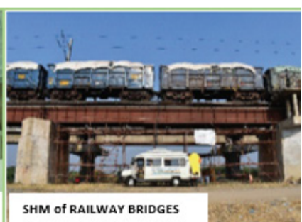
SHM of RAILWAY BRIDGES
