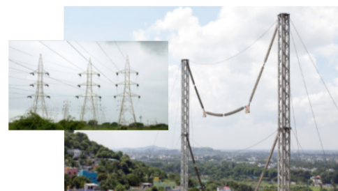
Emergency restoration system for power transmission line
