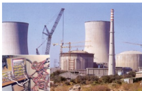
Condition assessment of power plant structures
