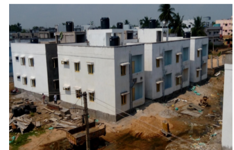
Light weight pre-fab construction for mass housing
